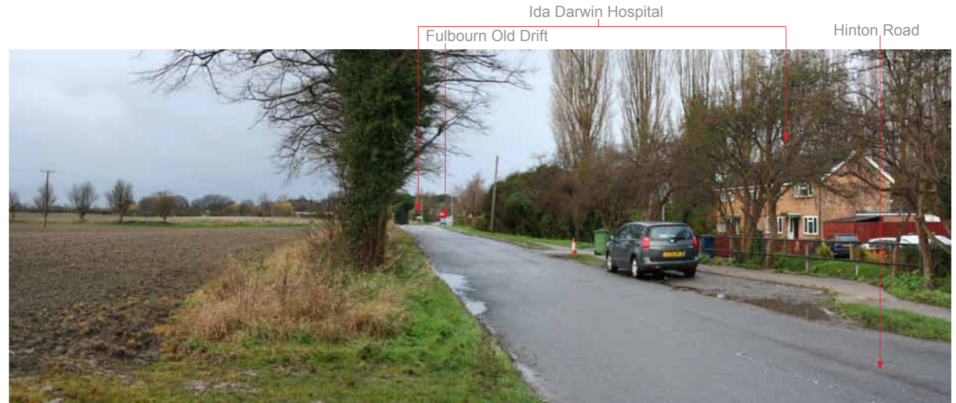
Westerly view from Hinton Road towards site
